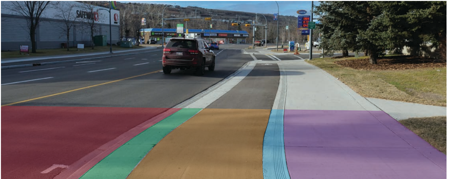
NEW BOWNESS ROAD CROSS-SECTION FOR ARTERIAL STREET SECTION, INCLUDING UNI-DIRECTIONAL CYCLE TRACK AND BUFFER ZONES
