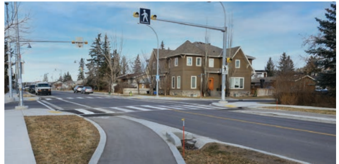
IMAGE 5. CURB EXTENSIONS AND DIRECTIONAL CROSSWALKS AT BOWNESS RD AND 43 ST INTERSECTION, AND ENHANCED PEDESTRIAN FLASHERS ON BOTH SIDES OF THE STREET
