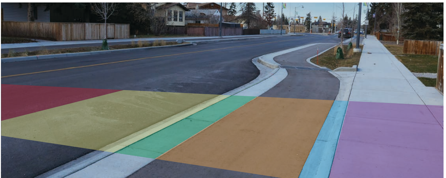
NEW BOWNESS ROAD CROSS-SECTION FOR NEIGHBOURHOOD BOULEVARD (RESIDENTIAL) SECTION, INCLUDING UNI-DIRECTIONAL CYCLE TRACK AND BUFFER ZONES
